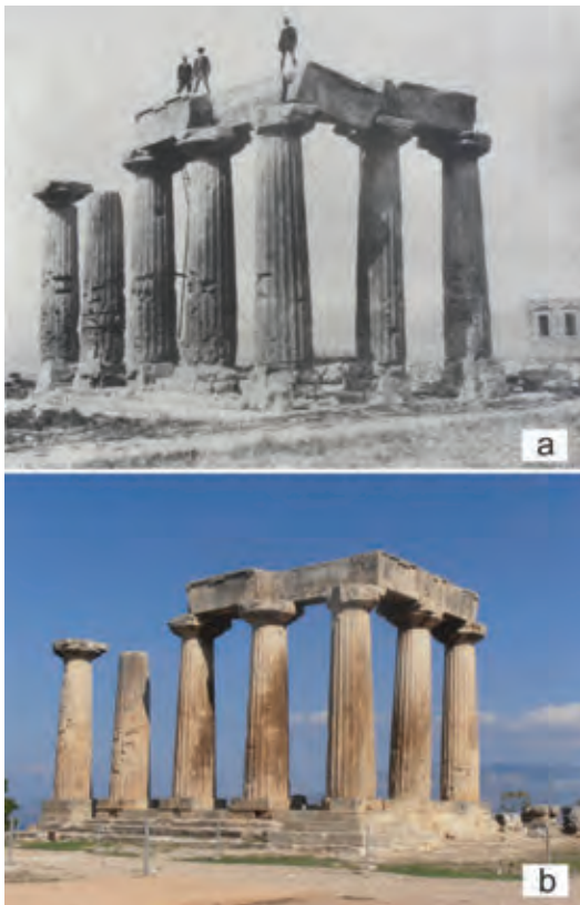
Figure 6: (a): The Temple of Apollo in 1901. Note the two metal rings that support the single fractured column without a capital, and the displaced outer corner epistyle. This figure is also indicative of the poor state of preservation of the temple base, (ASCSA Corinth Excavations). (b): The Temple of Apollo in our days with rescue restoration measures taken on the epistyle, the base and the fractured column).
