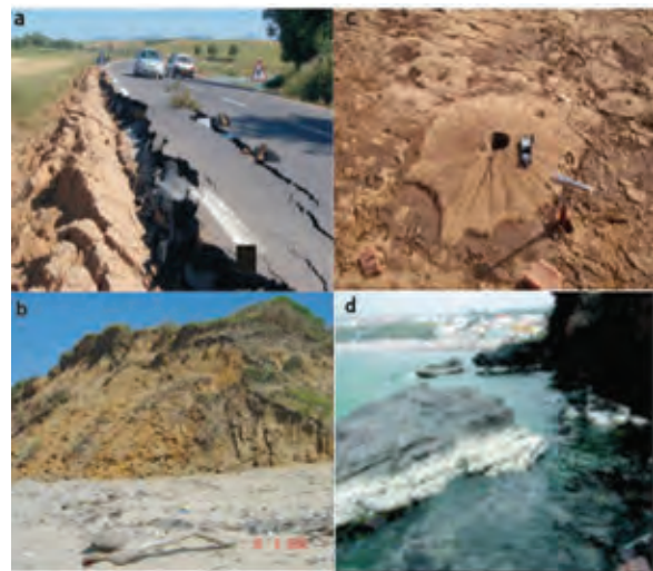
Figure 2: Ground effects observed after 2003 Boumerdes (Algeria) earthquake. a: cracks, b: slope movements, c: volcano crater of liquefaction, d: coastal uplift.
