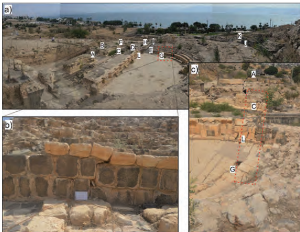
Figure 3: a) General view of the Berniki theatre (looking NE); the letters show locations of main features. b) Detail of an observed deformation. c) Alignment of deformations along a N140° direction.
