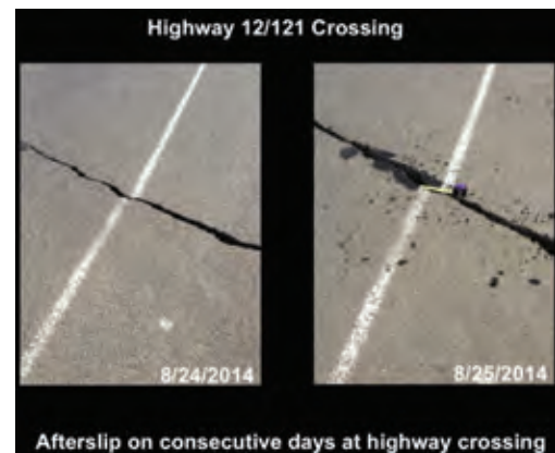
Figure 4. Afterslip across CA Highway 12 on the day of the earthquake (8/24/14) and on the day following (8/25/14). Afterslip was rapid and will approximate the amount of coseismic slip on the northern half of fault trace A. Photos by Tim Dawson, California Geological Survey.
