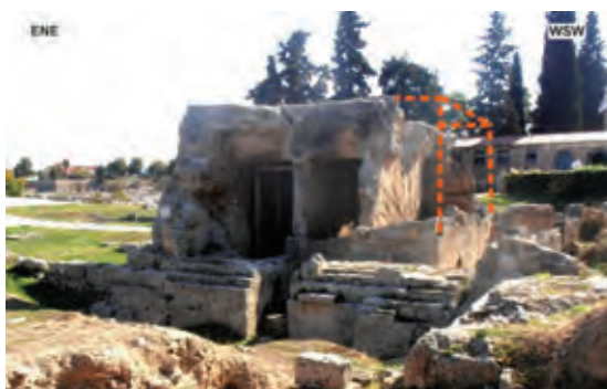
Figure 8: The NNW facade of the Glauke Fountain. With dashed line the section of the monument that collapsed during the earthquake of 1928.
