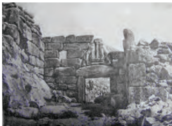
Figure 1: Mycenae, the Lion Gate before excavations and restoration (Tsountas 1893, fig. 3). The famous fault plane – which did not move for at least 3000 years – is on the lower left. Note the missing two ashlar right of the lion relief. The dressed exterior and rubble interior of the western wall on the right was still visible at that time.
