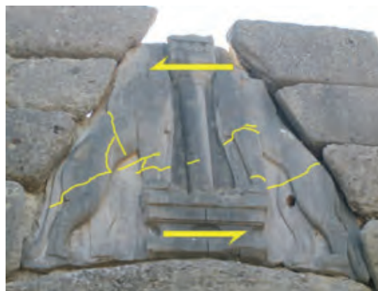
Figure 4: The lion relief. The monolith is 3.9 m wide, 3.3 m high and up to 0.7 m thick. A network of open fractures (marked by thin lines) across the relief is interpreted as caused by the hit of the two ashlars on the upper right side during seismic shaking. These two blocks fell to the ground and were still there in the 19th century as shown in Fig. 1. Apparent lack of continuity of the fracture on both sides of the half-column is due to thin, dark crust produced by blue-green algae. #1095.
