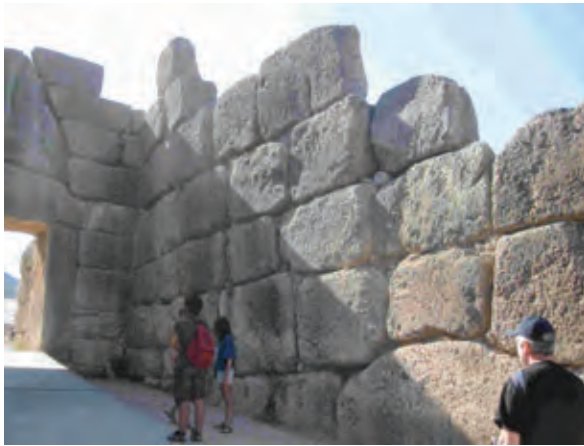
Figure 2: The western wall in the forecourt of the Lion Gate. There are eight rows of well-dressed ashlars, obviously not in the same plane. Top of the long wall is 6.85 m above ground level. People for scale. Photo Kázmér, #1097.
