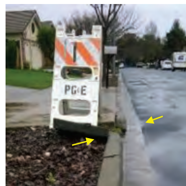
Figure 3: Distributed ground displacement associated with the 2014 Mw6 earthquake in the Napa valley, California. The curb is dextrally displaced of about 5-7 cm, associated with the Browns Valley strand.
