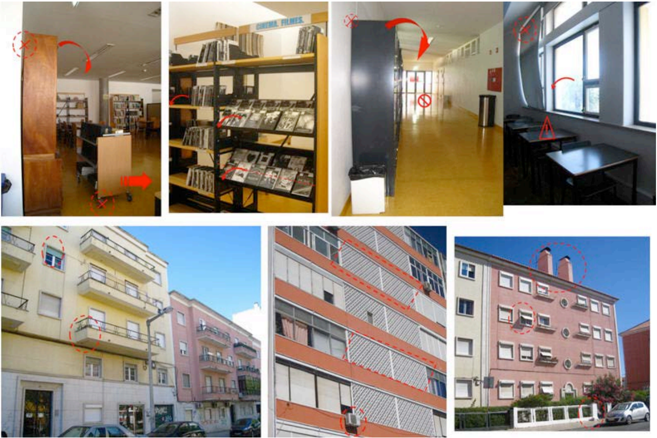
Figure 1. Identification of some non-structural components in the interior of schools and in housing stock of Alvalade (Portuguese pilot area).
