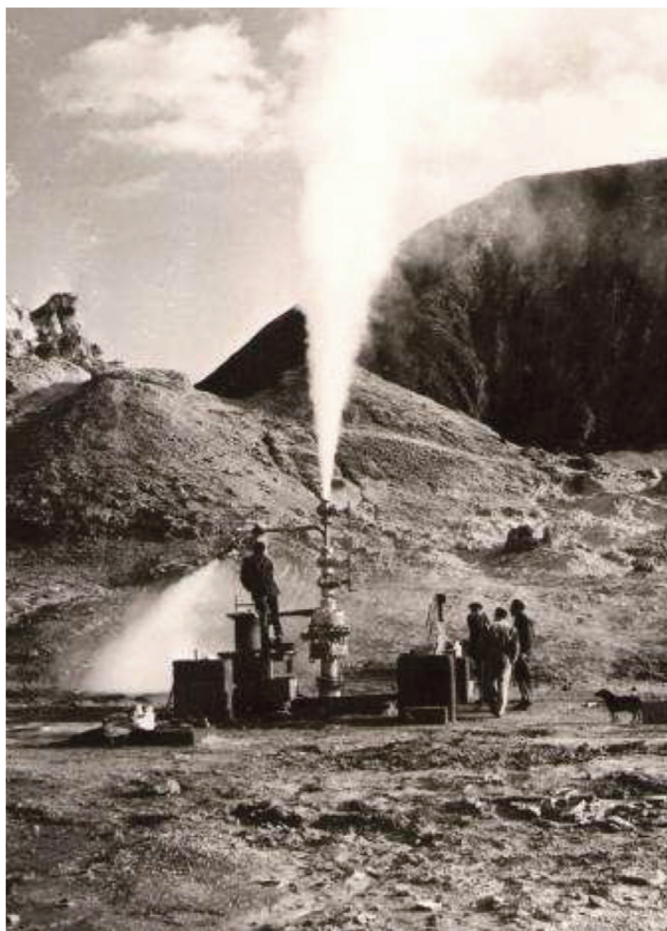
Figure 1 Drilling VU2bis at Vulcano island during the test for production of dry vapour in 1955 [from Sommaruga, 1984].
