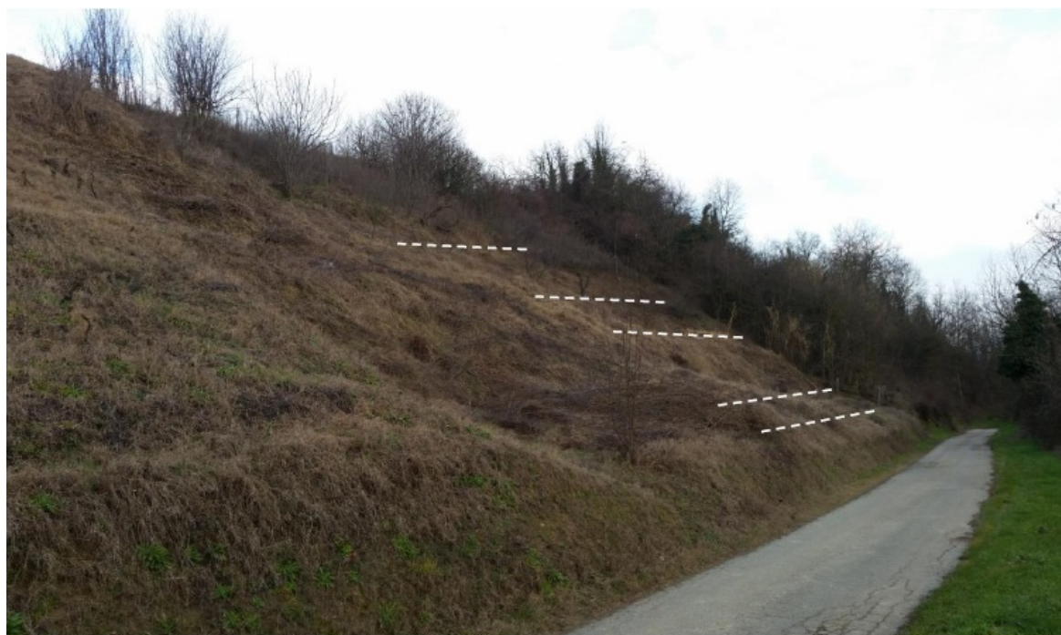
Figure 2. Arrangement of rotational slip with anthropic terraces, underlined by dotted lines, involving Ferrere Unit sediments on the right sector and recent rotational landslide on left sector.
